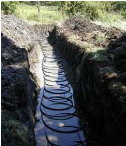
Figure 2: Installation of coiled GCHP
