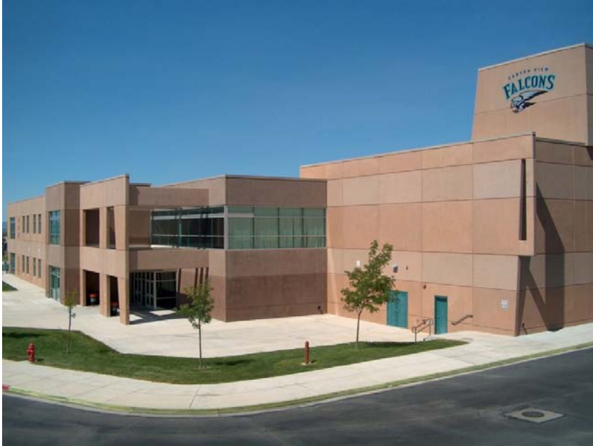
Figure 4: Canyon View High School, Cedar City, Utah
